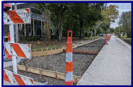
Carey Street Pavement Reconstruction
